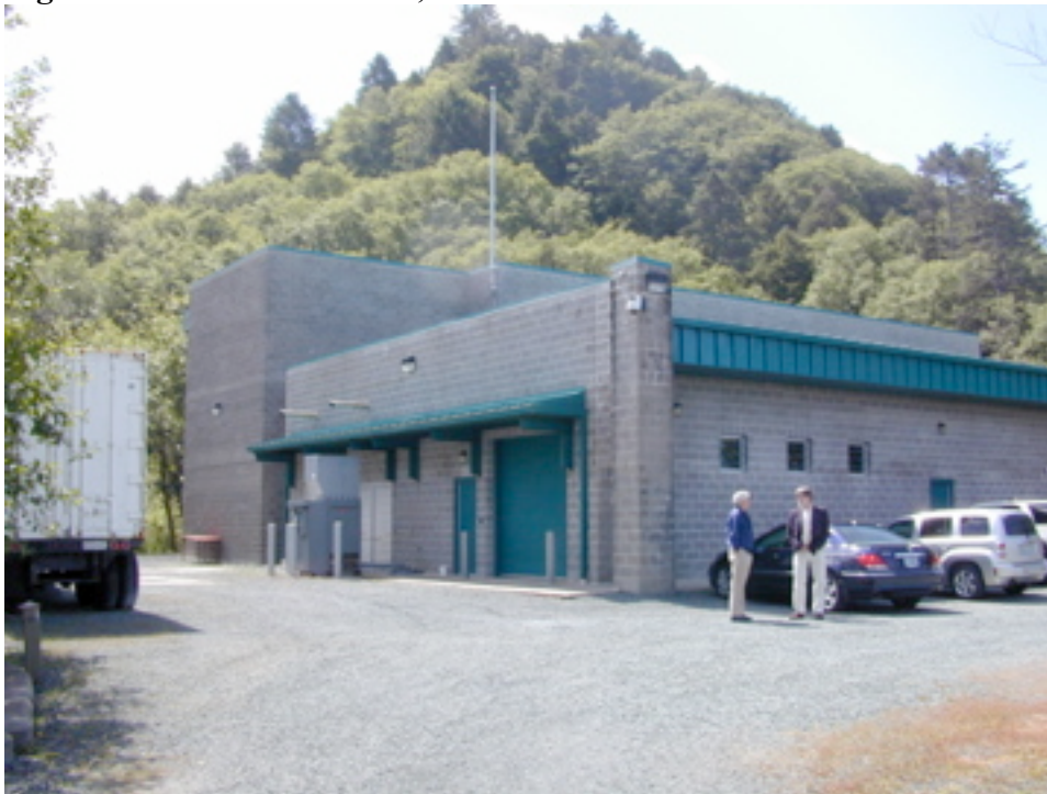
Figure 12. Nedonna Station, Exterior
